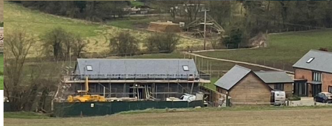
12 th January 2024 Roof on
