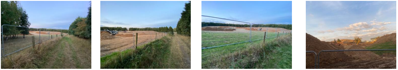
Above: 13 th September 2021 – 31 st January 2022 the progress of the warehouses can be seen on the right. In the field beyond the line of fir trees was the old Apple Shed.
