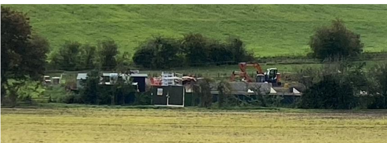
27 th September 2023 Piggeries demolished, front view from Somersham Road
